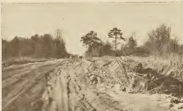
FIGURE 66.—DRY LAND FILL CONSTRUCTED ON GROUP A-8 SUBGRADE IN VIRGINIA
